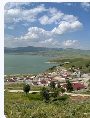
Alpaslan 2 HPP and dam (280 MW)
